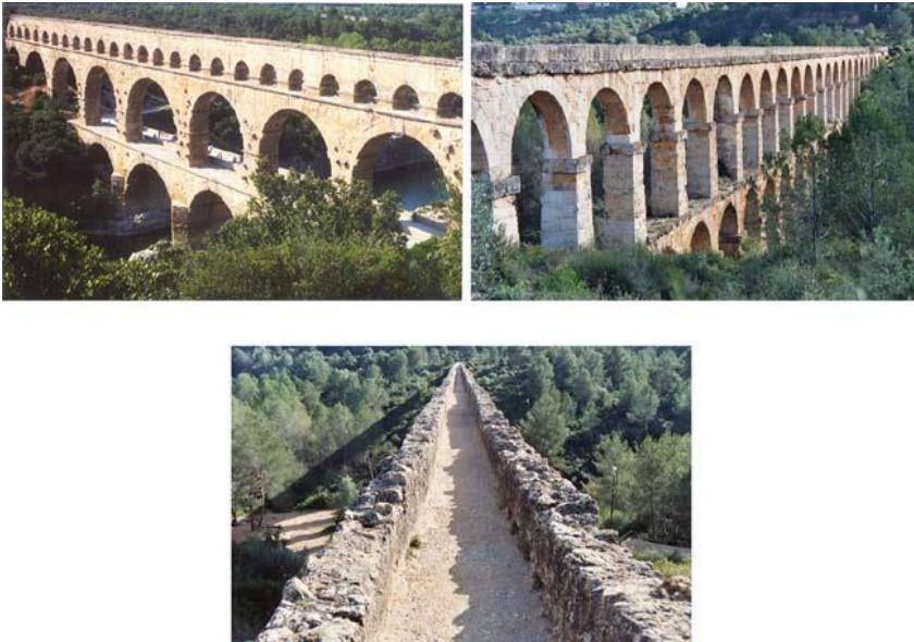
Fig. 2. Apeducte romane: a. Pont du Gard; b. Ferreras; c. Conductă de tip specus , Ferreras (Mays, Ancient Water Technologies , p. 119).
