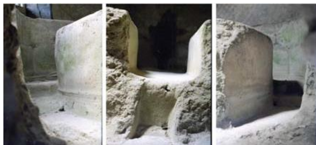
Fig. 6. Castellum divisorium , Pompei. a. Exterior; b-d. Interior (după Mays, Ancient Water Technologies , p. 122).
